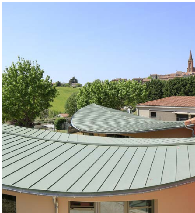
Standing seam roofing VMZINC® - PIGMENTO® lichen green - Architect: Bamboo - Caraman - France
