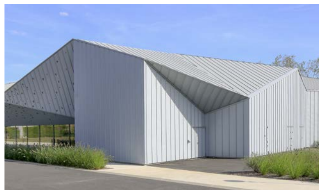
Standing seam roofing VMZINC®, Perforated sheets - PIGMENTO on request - Architect: Vignault x Faure - Pornic - France
