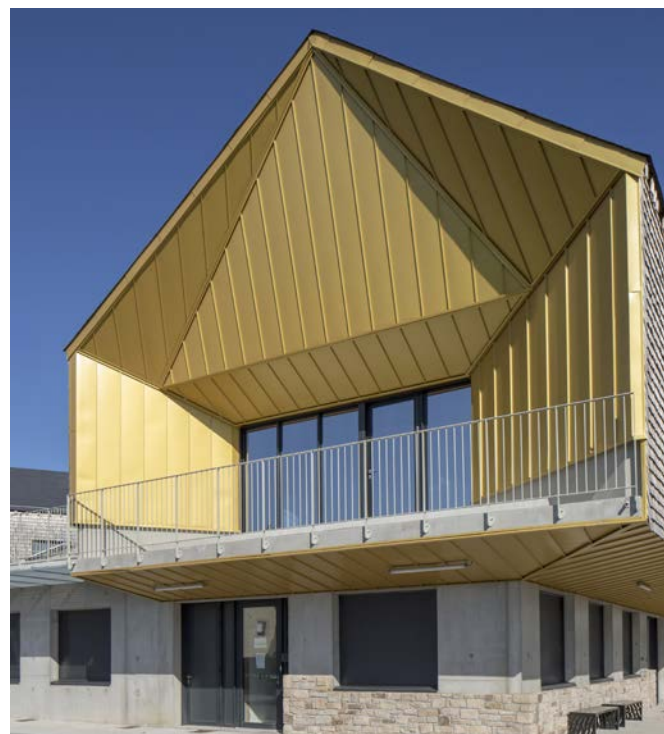
Standing seam roofing VMZINC® - PIGMENTO on request - Architect: Vignault x Faure - Crac'h - France
